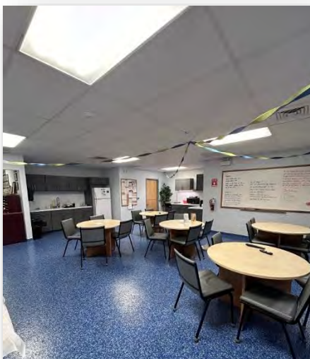
New Kitchen Cabinet and Floor
