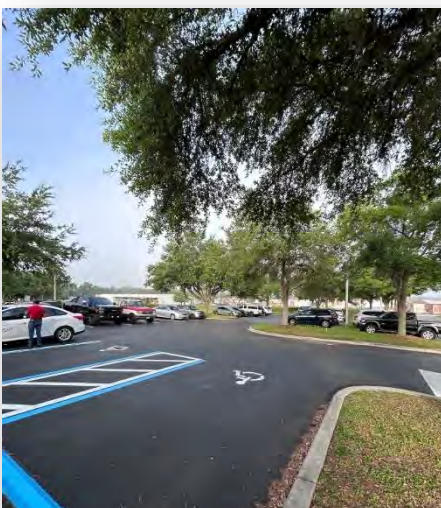
Renovated Parking Area
